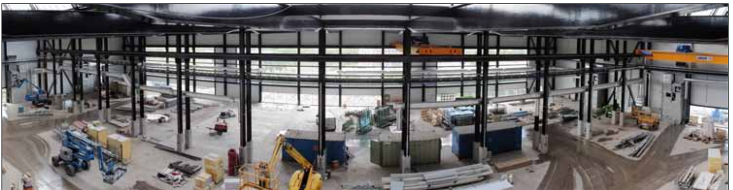
The Nuclear AMRC workshop covers the area of four Olympic swimming pools. The largest machining centres to be installed weigh up to 80 tonnes apiece.
